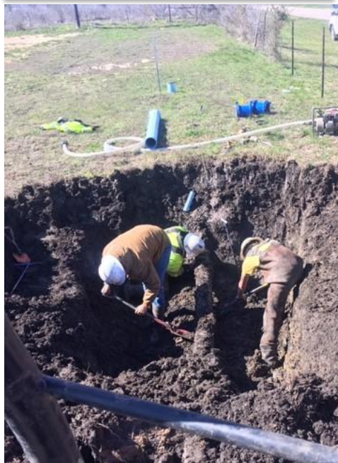
Leak repair above
